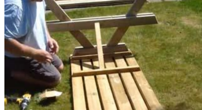
Put into place the trestle support
