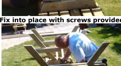
Fix next A-frame trestle into position
