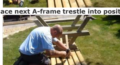
Put & fix into place trestle support
